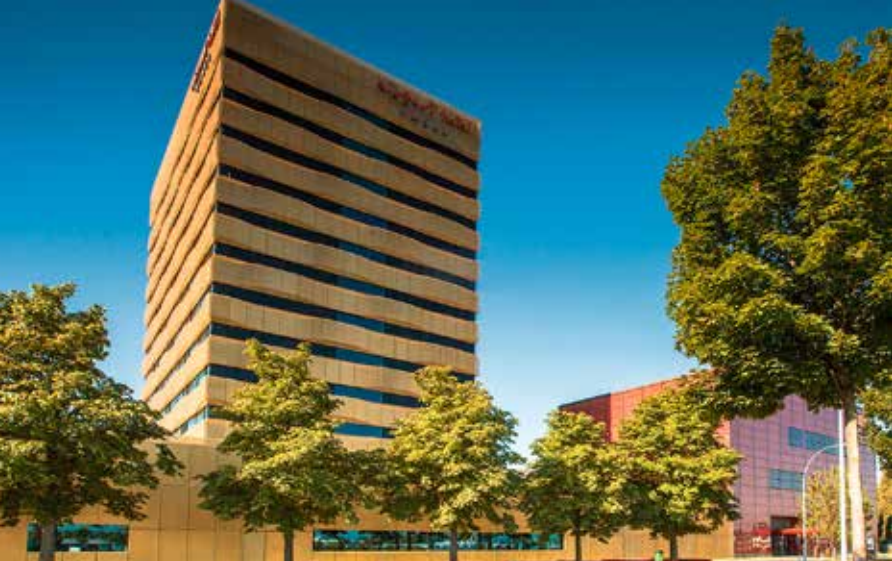
Airport Hotel Basel
