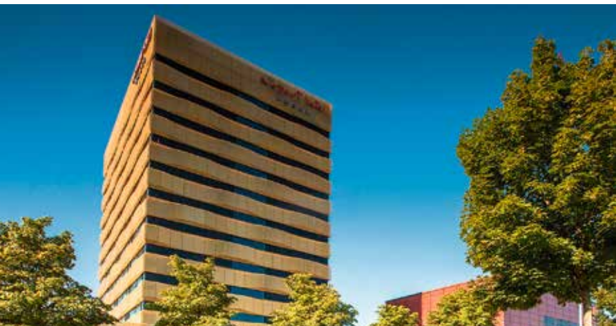
Airport Hotel Basel
